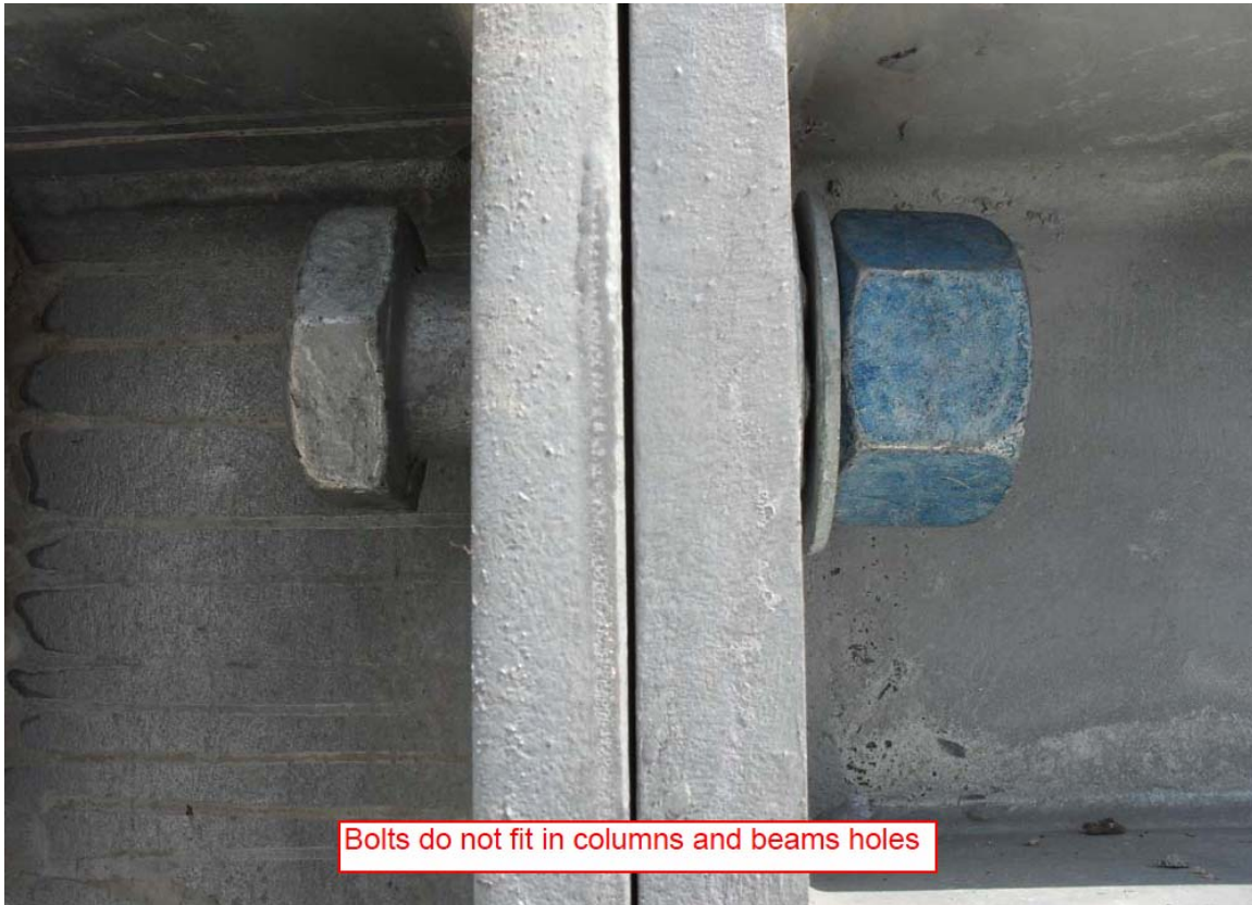
Photo courtesy of Fluor Constructors, Inc.
