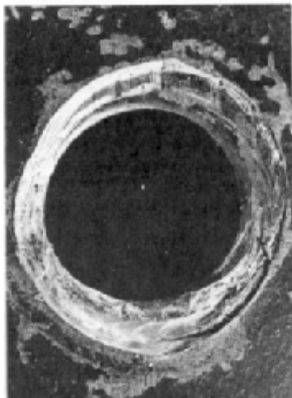
Fig. 9.3. Severe galling of plate under turned element (1/4 in. clearance, no washer).
