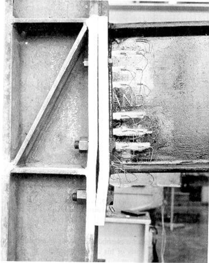
Fig. 18.16. End-plate after failure. (Courtesy of University of Sheffield.)
