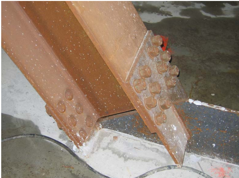
Figure 1.1 Shear connection in a bracing member
